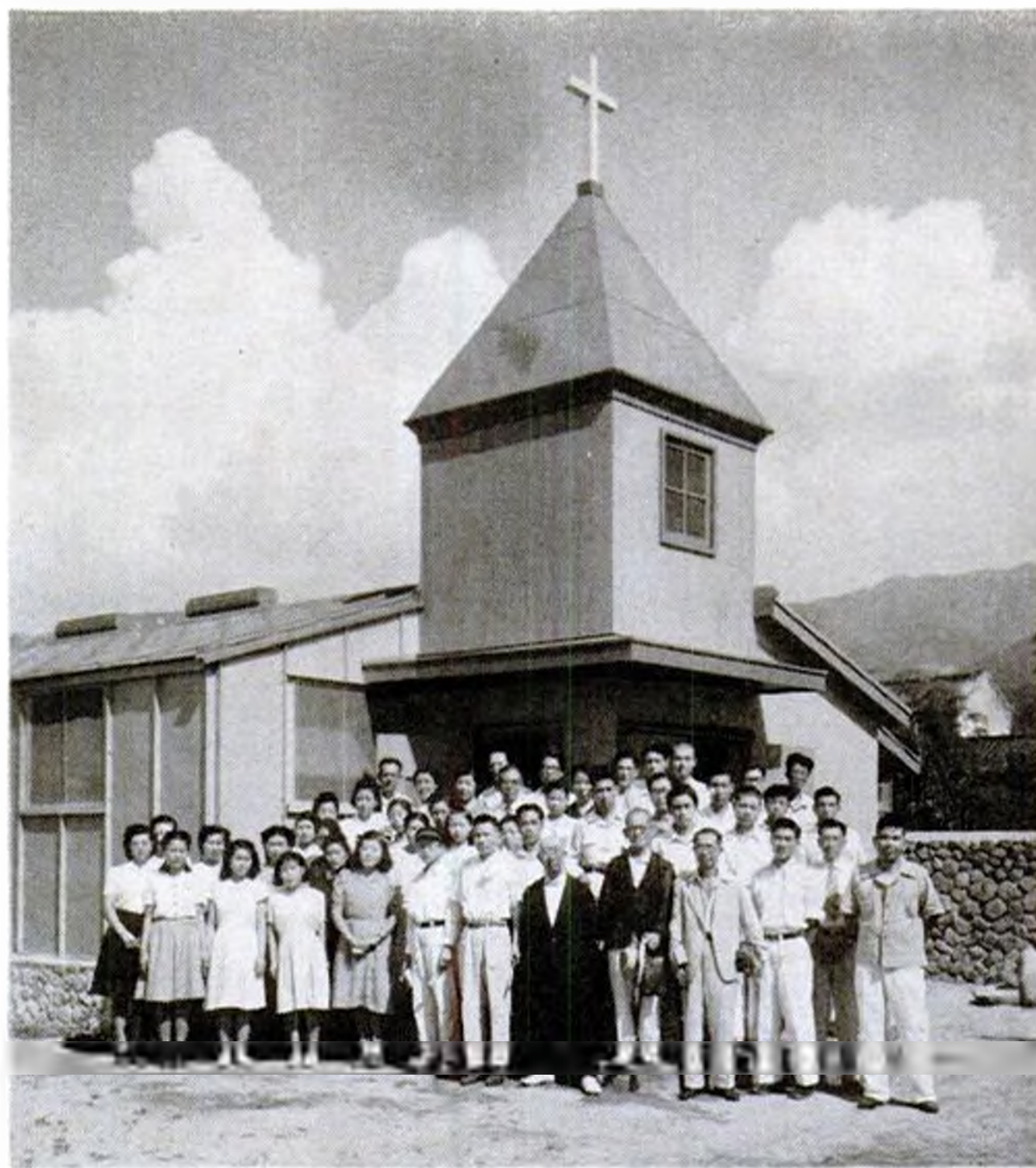
PREFAB ALUMINUM CHURCH IN KOBE SERVES A SMALL CONGREGATION
